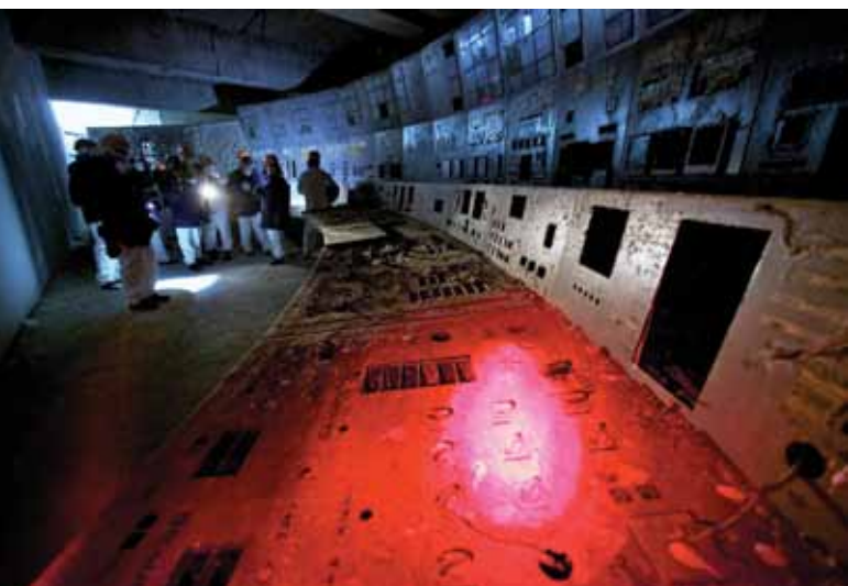
The control room of the stricken Chernobyl #4 reactor.
