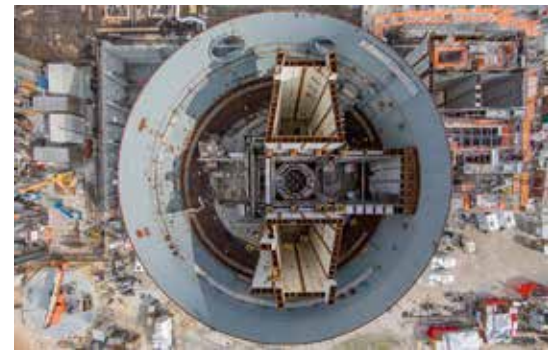
The Vogtle #4 reactor under construction in Georgia.
